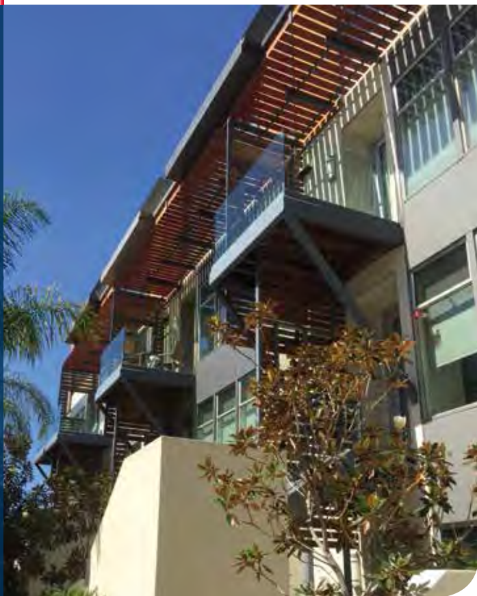
KNX installation in the home in Los Angeles
